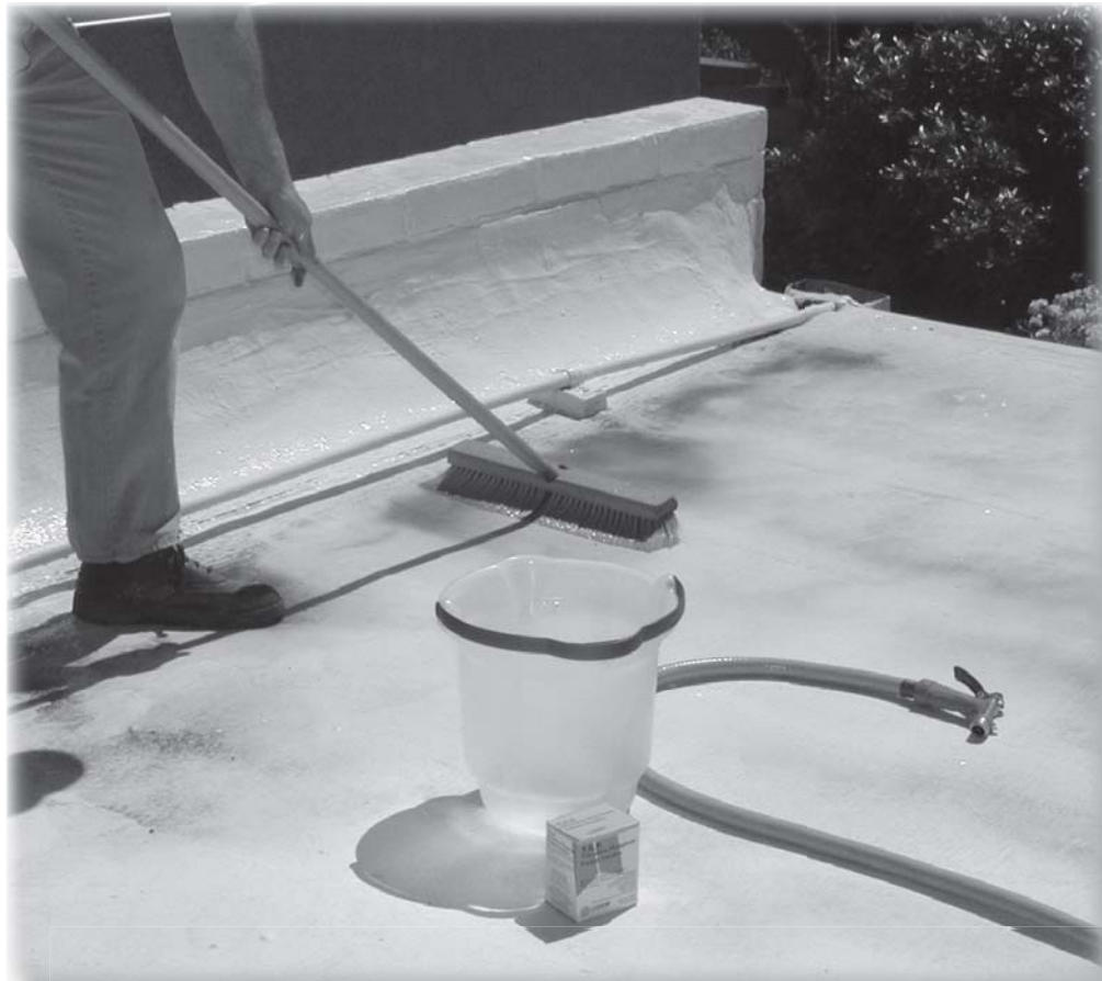
Regularly cleaning a roof during its lifetime will maximize energy savings from reflectivity.
