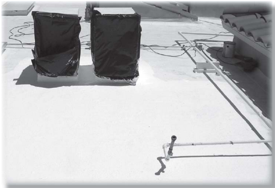
At least one local contractor will pressure wash and coat the placement area with Solar Tek Extreme as a regular part of the job. Above you can see the dramatic difference.
