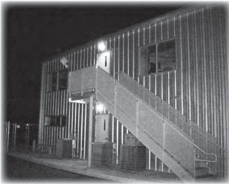
Late-working employees now have access to safely lit exits.
